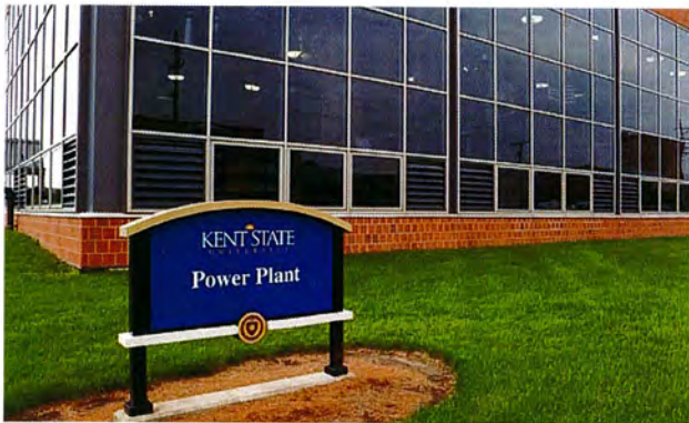
University Combined Heat and Power Energy Star Award
